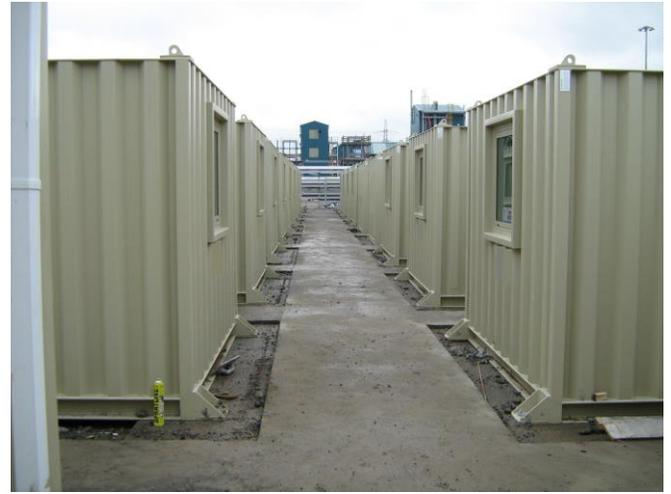
Ultrablast units are engineered to withstand a force of upto 1000-millibar over pressure for 100 milliseconds – the equivalent of exerting an 80 ton impact
